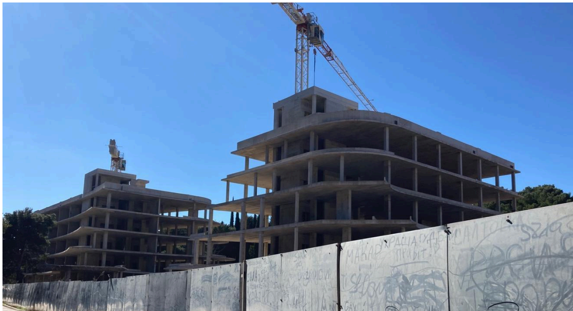
View of the structure of the condo hotel
