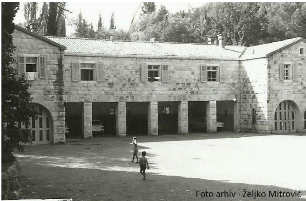
Royal garage demolished to build the condo hotel.
